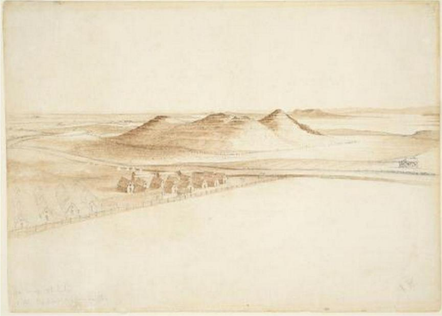
Figure 3. July 1861 drawing by John Kinder looking west to Mount Richmond from the McClelland Hills. Note the fencing around the base of the maunga and the lack of trees. From Grenfell 2015.
